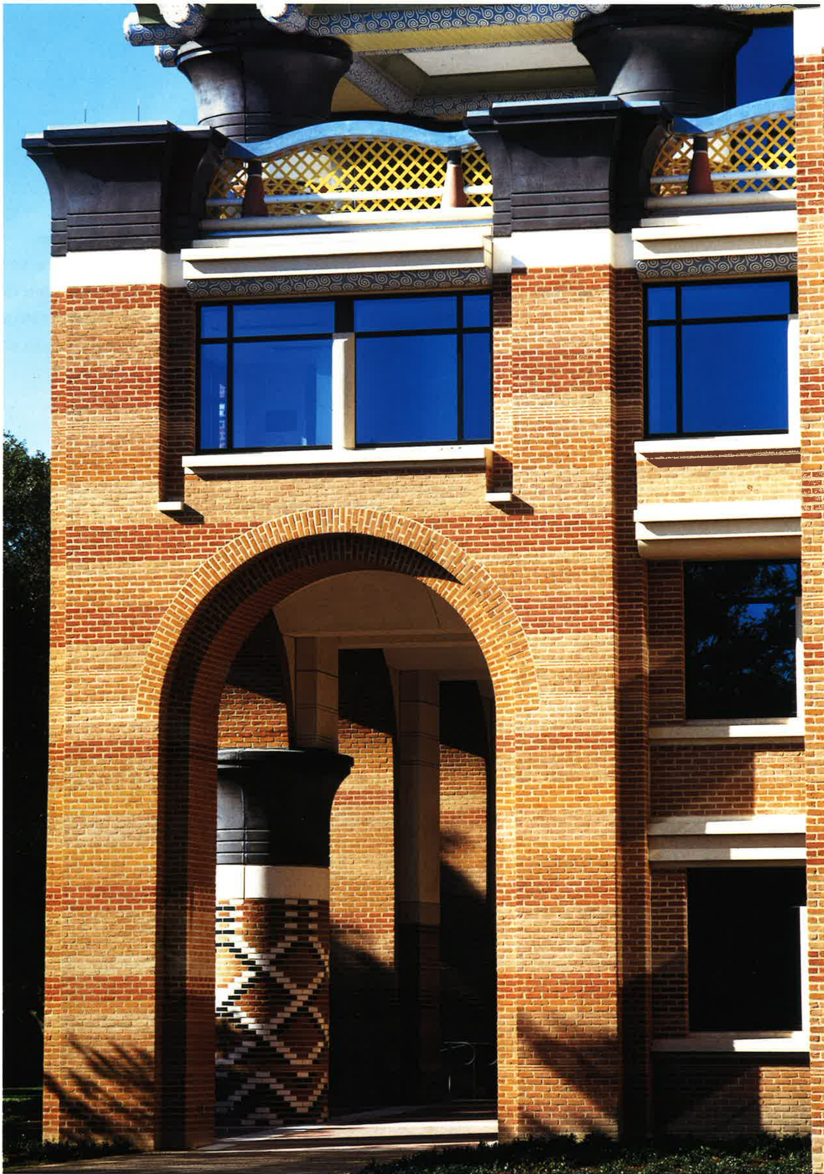
Computational Engineering Building, Rice University (Texas)
